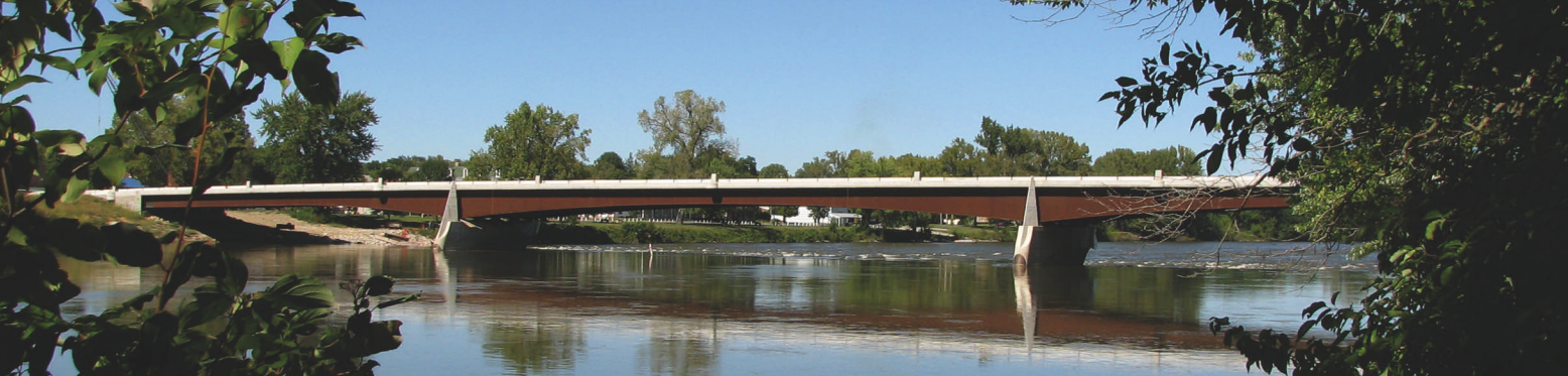
The bridge includes a 32-ft-wide roadway, a 5-ft-wide sidewalk, and a 10-ft-wide bicycle path.
