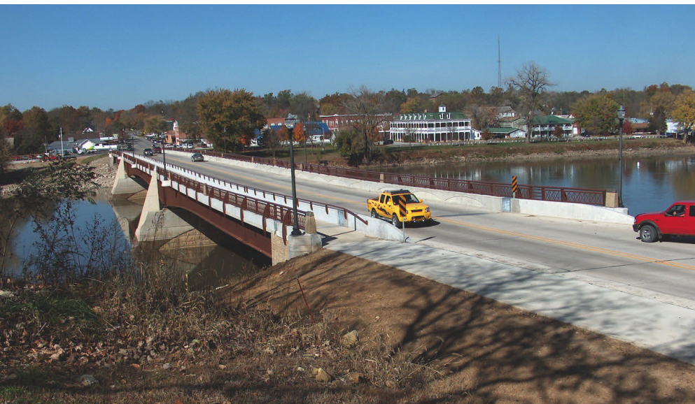
The bridge includes a 32-ft-wide roadway, a 5-ft-wide sidewalk, and a 10-ft-wide bicycle path.
